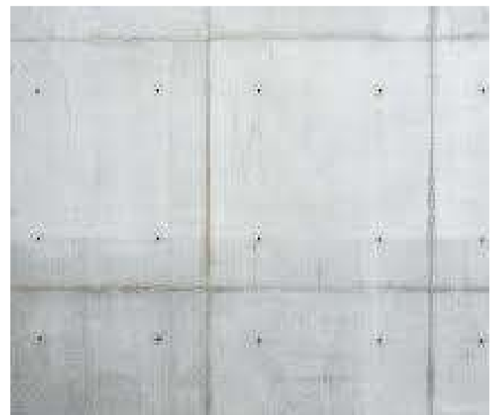
COF1 OFF-FORM CONCRETE WALL
